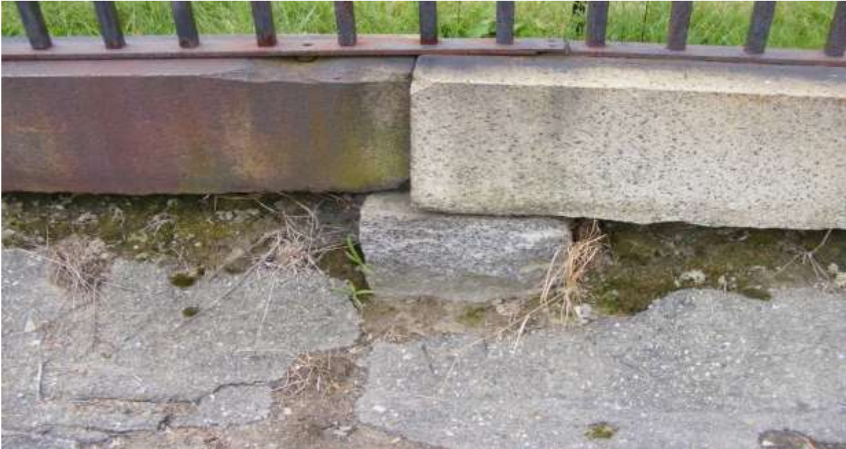
Cemetery Enclosure Fence and Stonework: Exposed wall support masonry
