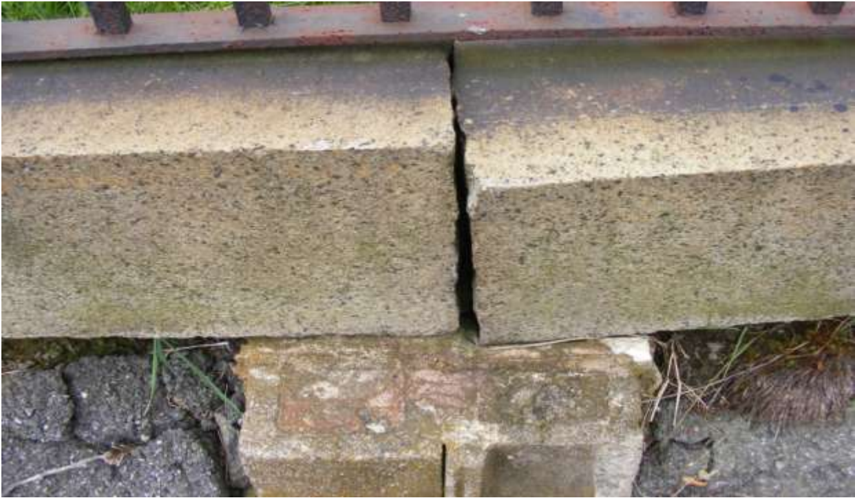
Cemetery Enclosure Fence and Stonework: Exposed wall support masonry
