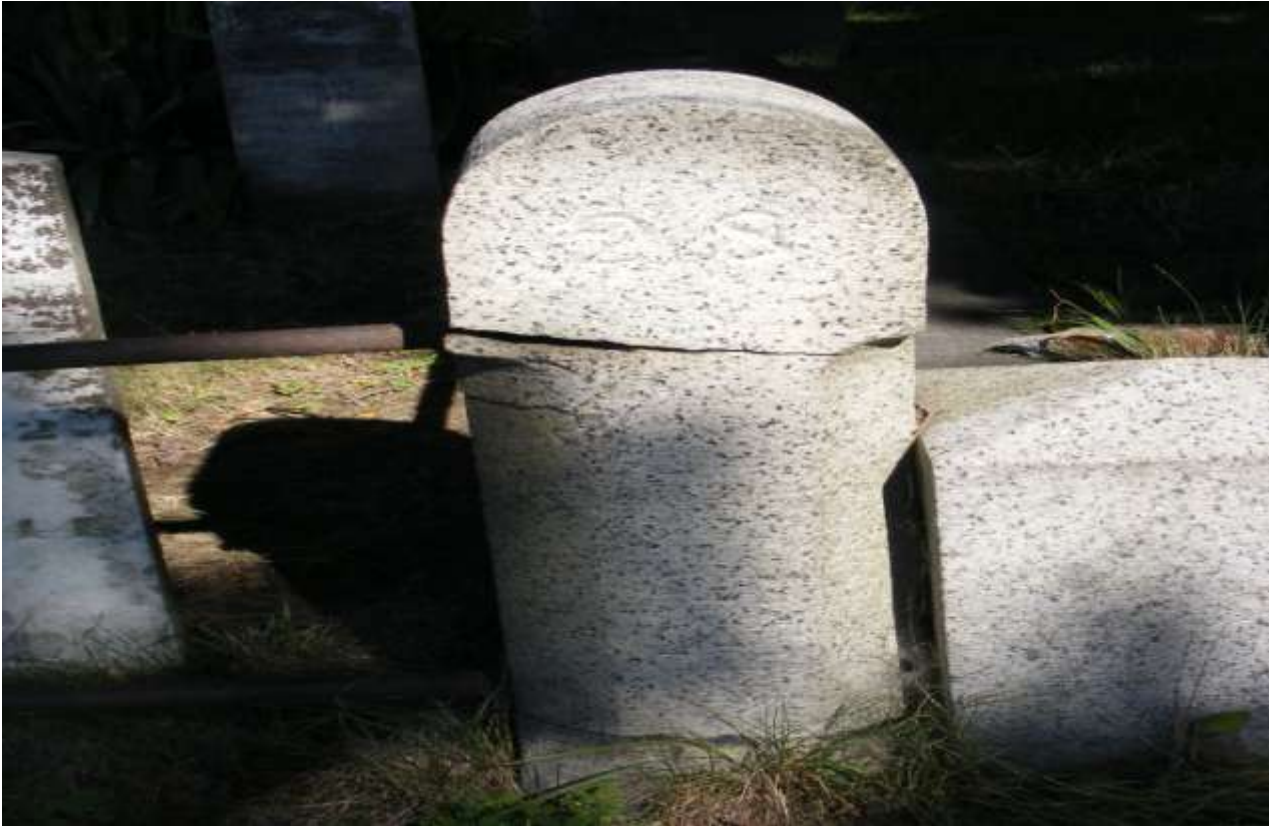
Granite Posts: Damage caused by expansion of rusted iron fence rail
