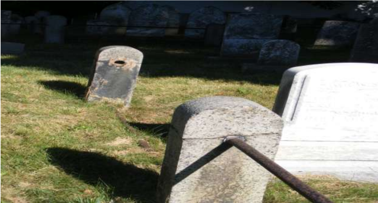
Granite Posts: Damage caused by expansion of rusted iron fence rail
